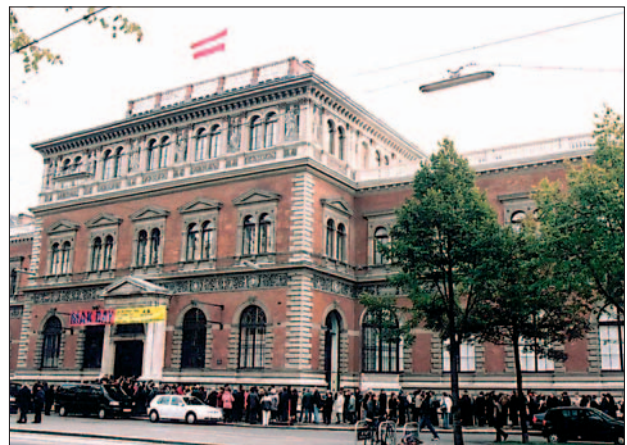
MAK DAY. Tag der offenen Türen, Haupteingang Stubenring
