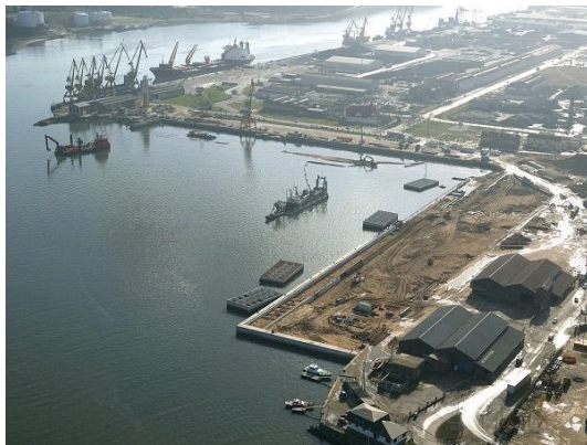
Situation during construction
