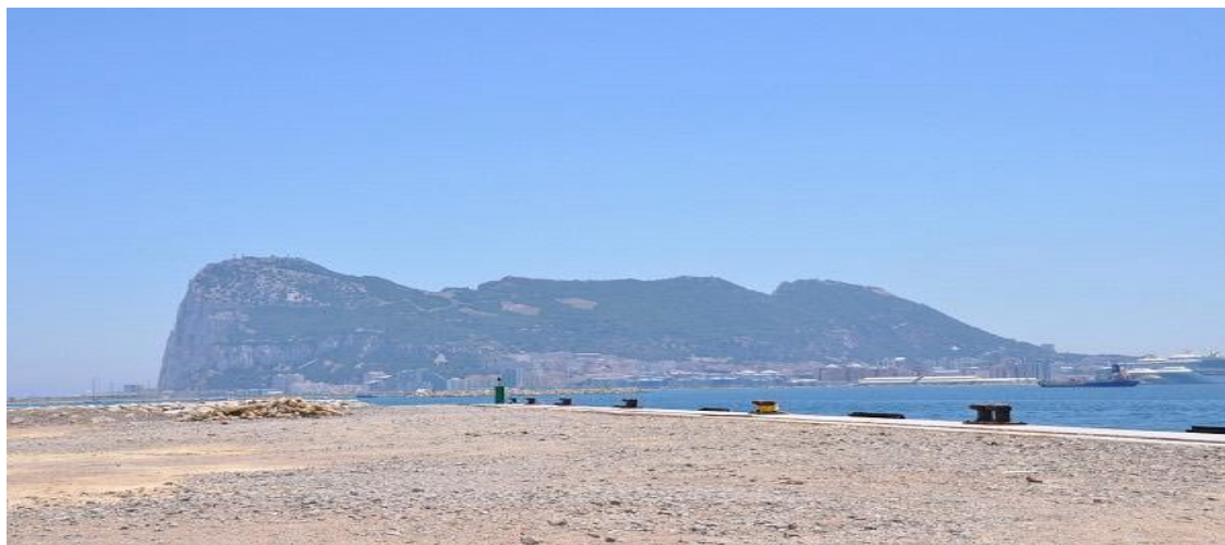
Part of the dock built in Campamento.
