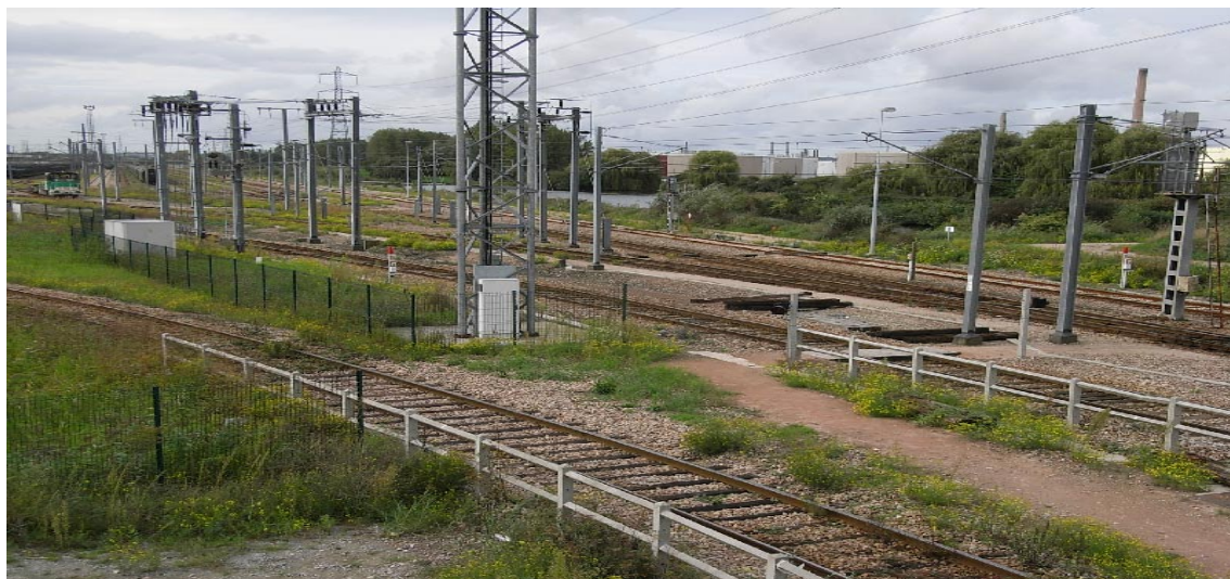
Part of the rail project co-funded in Le Havre.
