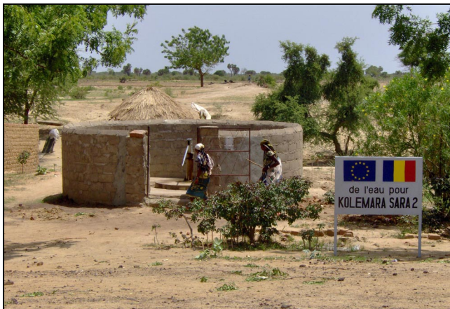
Waterhole construction in Kolemara Sara, Chad
