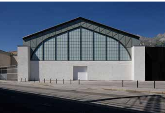
Innsbruck, Ing.-Etzel-Straße 31, Messehalle B © Hanspeter Schiess, Trogen/Schweiz
