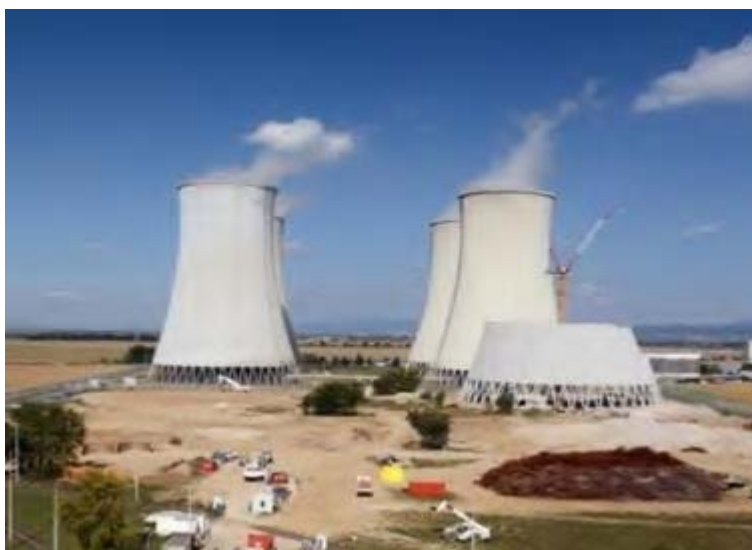
Figure 3 - Demolition of cooling towers.
