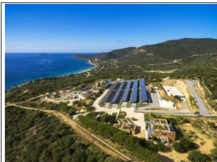
*The MYRTE and PAGLIA ORBA platforms in Corsica, France have been co-financed by the European regional development fund. These platforms produce and store energy through a hydrogen chain. This consists of an electrolysis apparatus which, during hours of low consumption, produces hydrogen and oxygen from water molecules. This energy is then distributed via a fuel cell producing electricity during hours of high consumption, for example in the evening, while the photovoltaic panels are inactive.*
