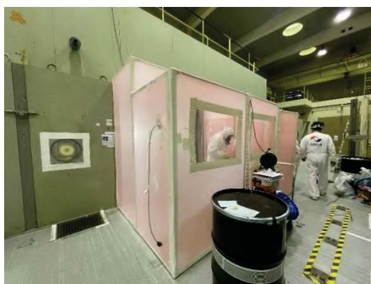
Ispra-Decontamination of hot cells in LCSR
