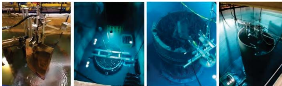
Figure 3: Cutting of Reactor Pressure Vessels at Bohunice
