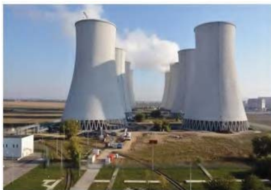
Before demolition of 4 cooling towers (09/2017)
