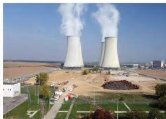
After demolition of 4 cooling towers (10/2018)
