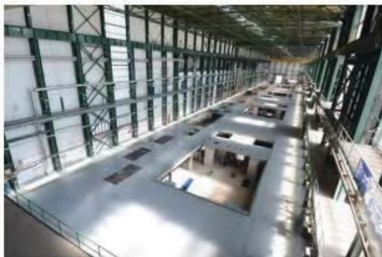
Turbine hall after dismantling (11/2016)
