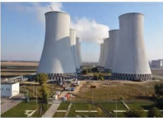
Before demolition of 4 cooling towers (09/2017)
