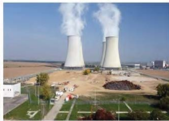
After demolition of 4 cooling towers (10/2018)
