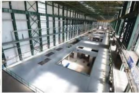
Turbine hall after dismantling (11/2016)
