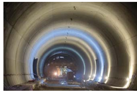
Tunnel T1 during construction
