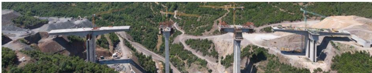
Bridge B3 during construction
