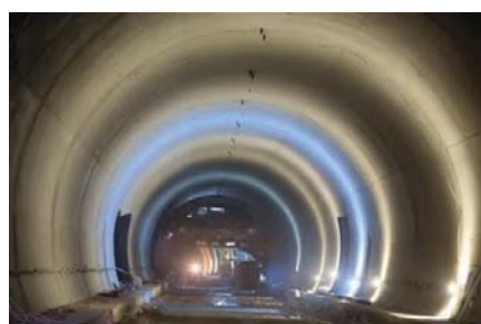
Tunnel T1 during construction
