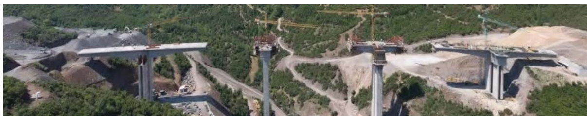
Bridge B3 during construction
